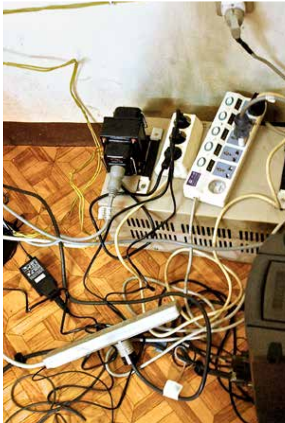
Dangerous equipment has been identified in some external reviews.
