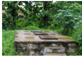
Figure 3 Protected pits with concrete covers, Nepal
